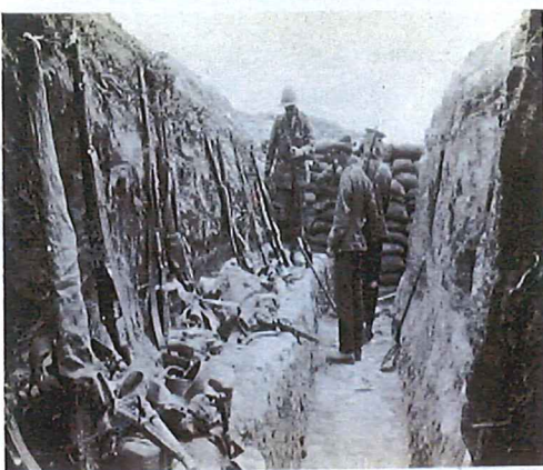
Last line reserve trench, men have moved back to give photographer clear view.
