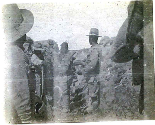
Gurkhas on fatigue improving communication trench. This lot were wiped out by J.J 5 mins after this was taken. This is only 20 yards from firing line where I was.
